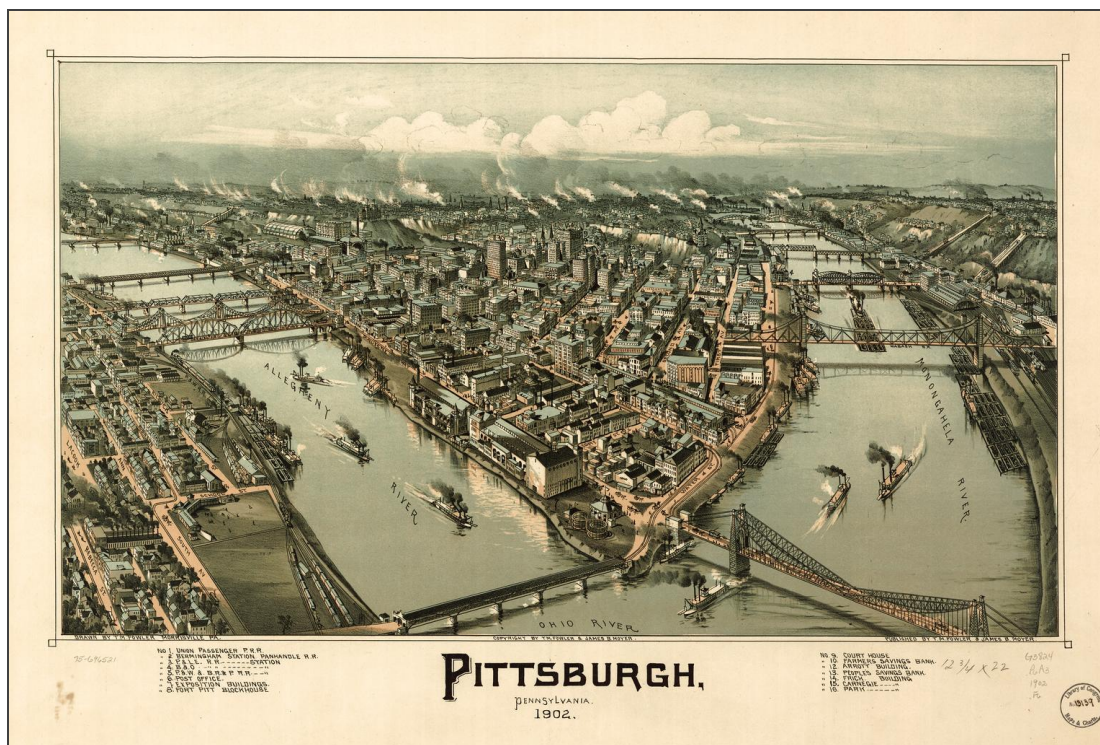
Panorama of Pittsburgh in 1902 showing the many bridges on the Allegheny and Monongahela Rivers
