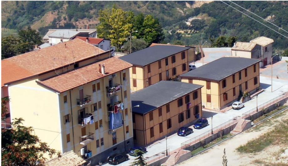
New area in Patricello (Aiello) where on October 27 th 1907 new homes were ready to be occupied by Aiellese homeless residents after the earthquake of September 8 th 1905. The construction of these homes was financed by the Veneto-Trentino and Milanese Pro-Calabria Committees .
