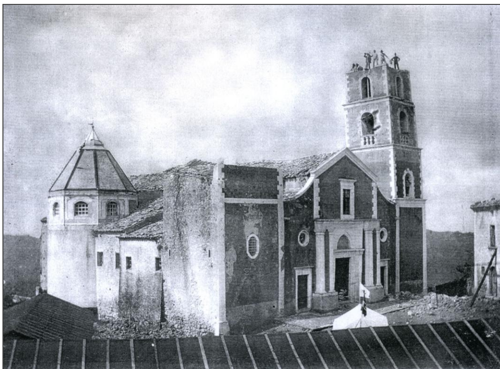
Church of St. Mary Major in Aiello: demolition of its steeple following the 1905 earthquake
