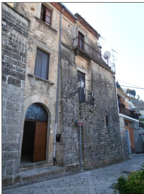
Palazzo De Dominicis Palace ) with a XVI century baroque balcony and in the entrance hall, a double flight of stairs with decorated stones (photo by F. Gallo)
