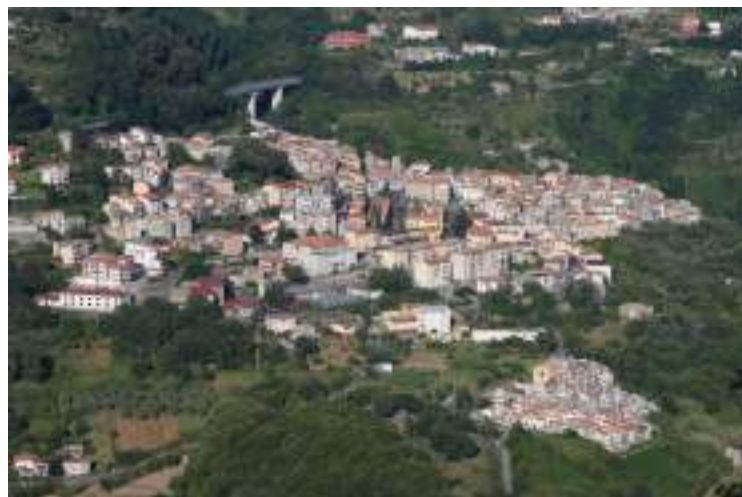
Lago: Cimitero sotto a destra Lago: its Cemetery at the lower right corner
