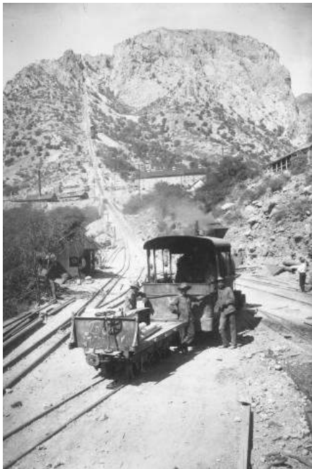
Coronado Incline Mine in Morenci, 1920
